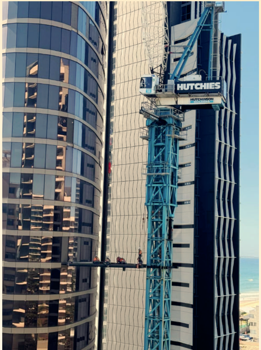
Riggers working to dismantle the crane on Royale Gold Coast.
