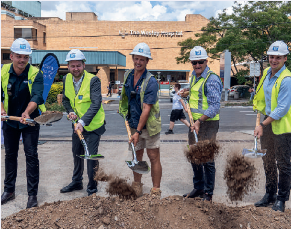
Hutchies’ team members helped turn the first sod to mark the beginning of construction on The Wesley Hospital project (from left) Isaac Andrasescu, Jack Hutchinson Jnr, Matt Grieves, Francois Pousson and Ethan Rosin.
