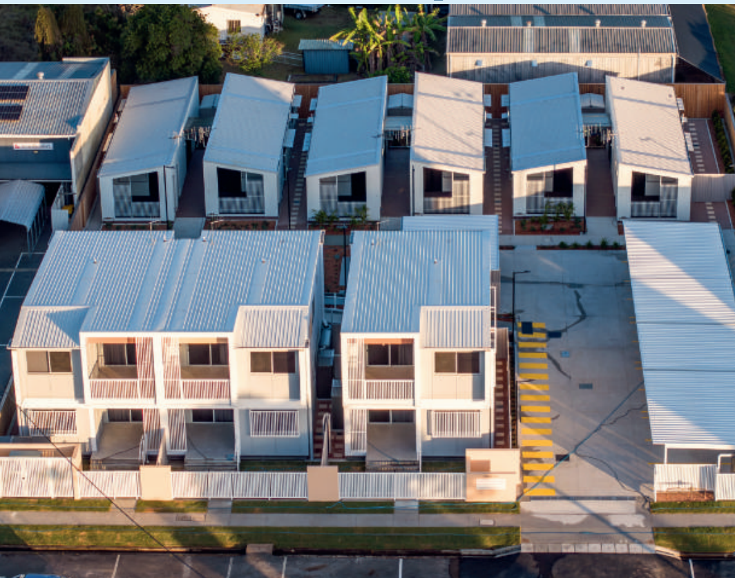
New low-rise residential development by Hutchies in Bundaberg East.
