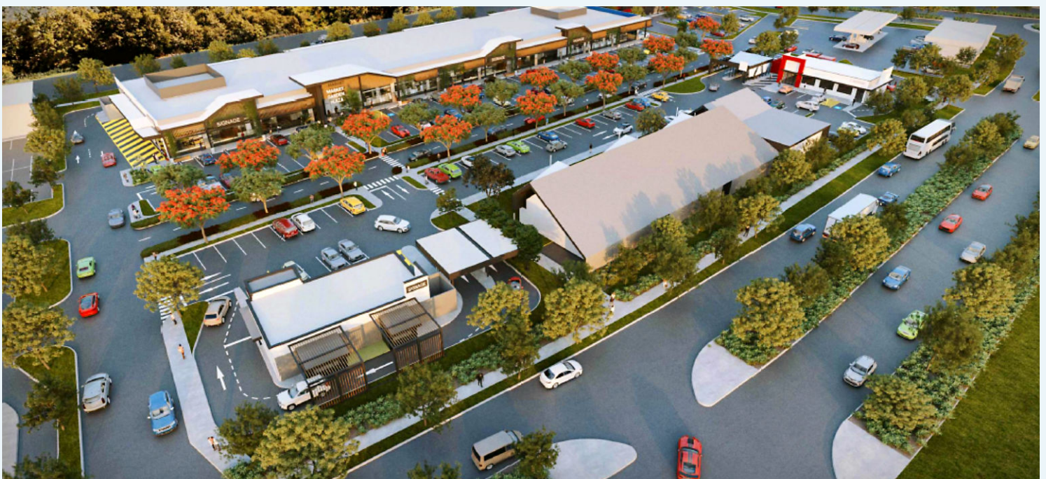
Townsville North Shore – a new mixed-use retail centre under construction by Hutchies.
