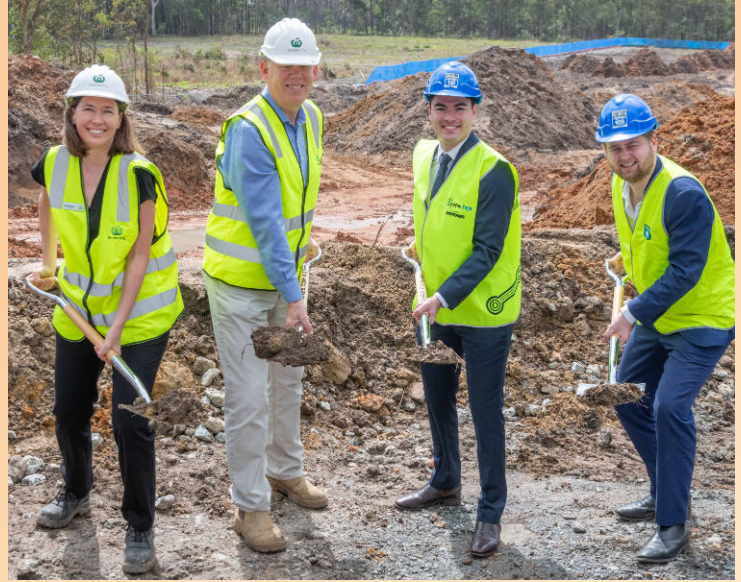
Sod-turning for Woolworths Logan Reserve Neighbourhood Shopping Centre in October (from left) Woolworths' regional development manager, Savannah Powell; Federal Member for Forde, Bert van Manen; Logan City Councillor, Jacob Heremaia; and Jack Hutchinson Jnr.
