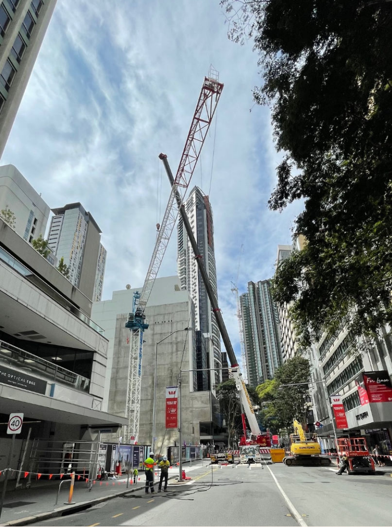
Installation of Hutchies' tower crane at 360 Queen Street, Brisbane.
