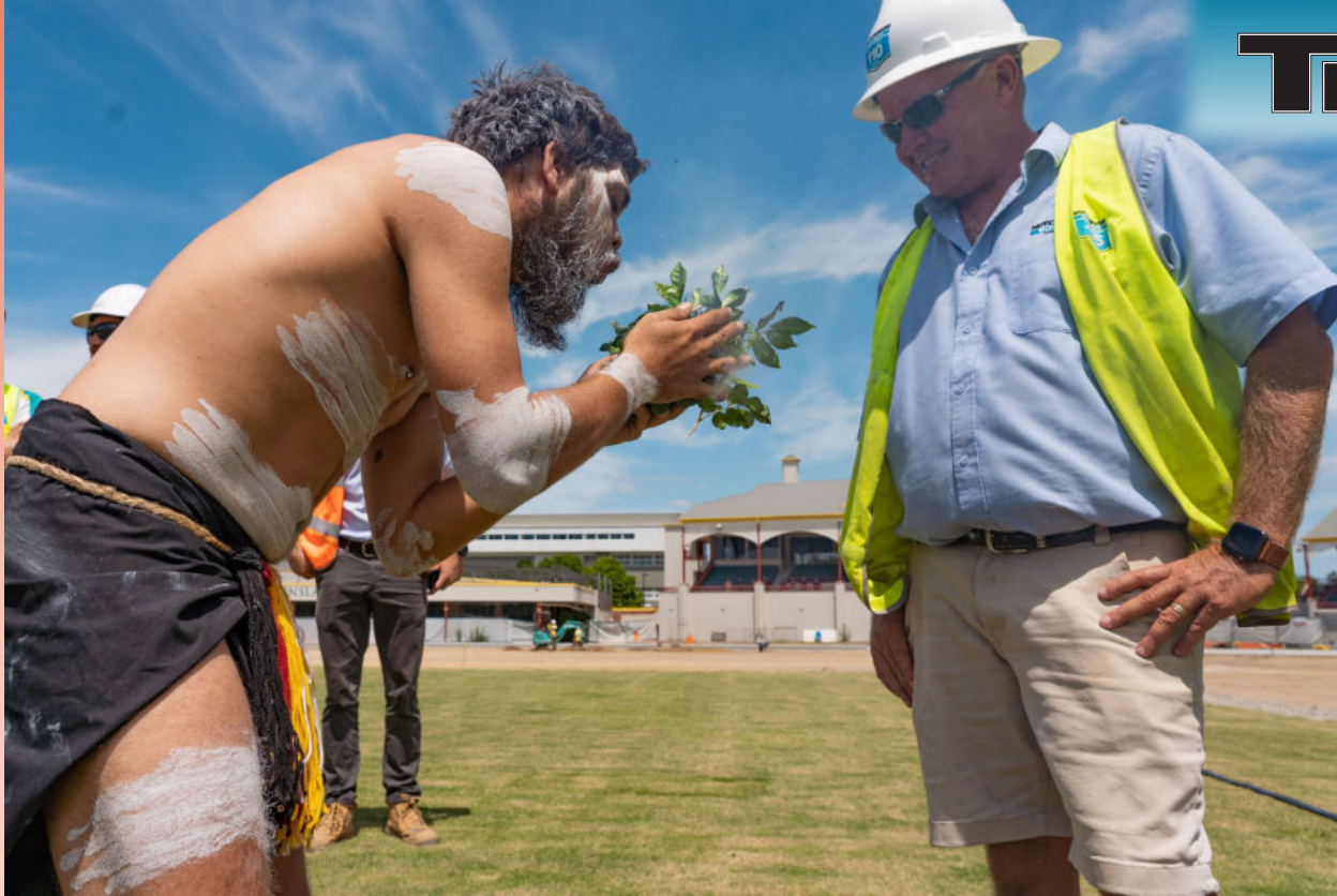
LEFT: Hutchies' site manager Dan Staples joins in the smoking ceremony at the Allan Border Field redevelopment project.
