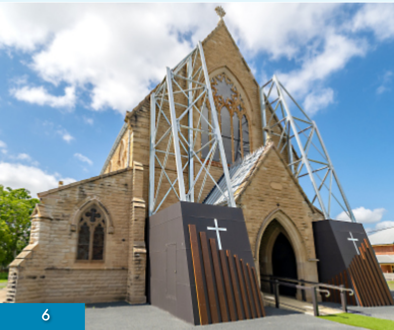
LEFT: St Paul's under repair showing the temporary steel props.
