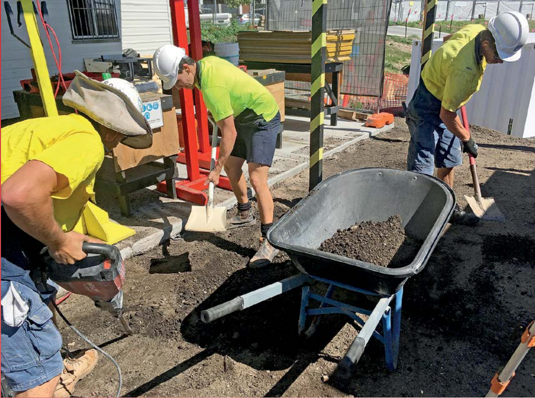
Apprentices busy at work during the concreting workshop.
