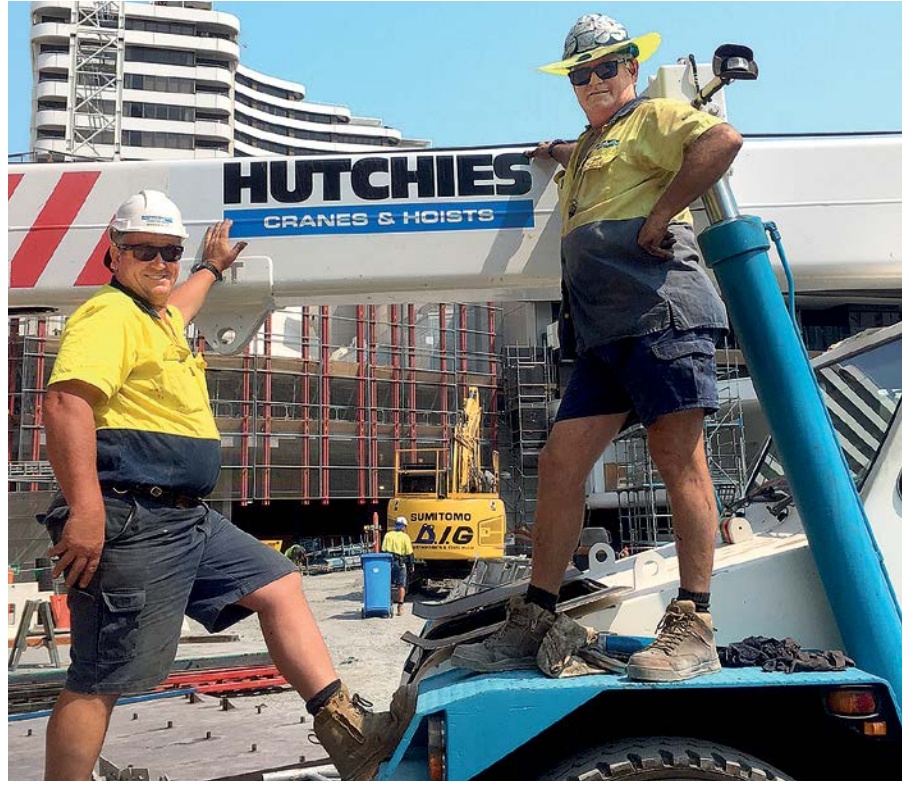
Greg Whitbread (left) and Donny McKenzie with Hutchies Cranes and Hoists' equipment.
