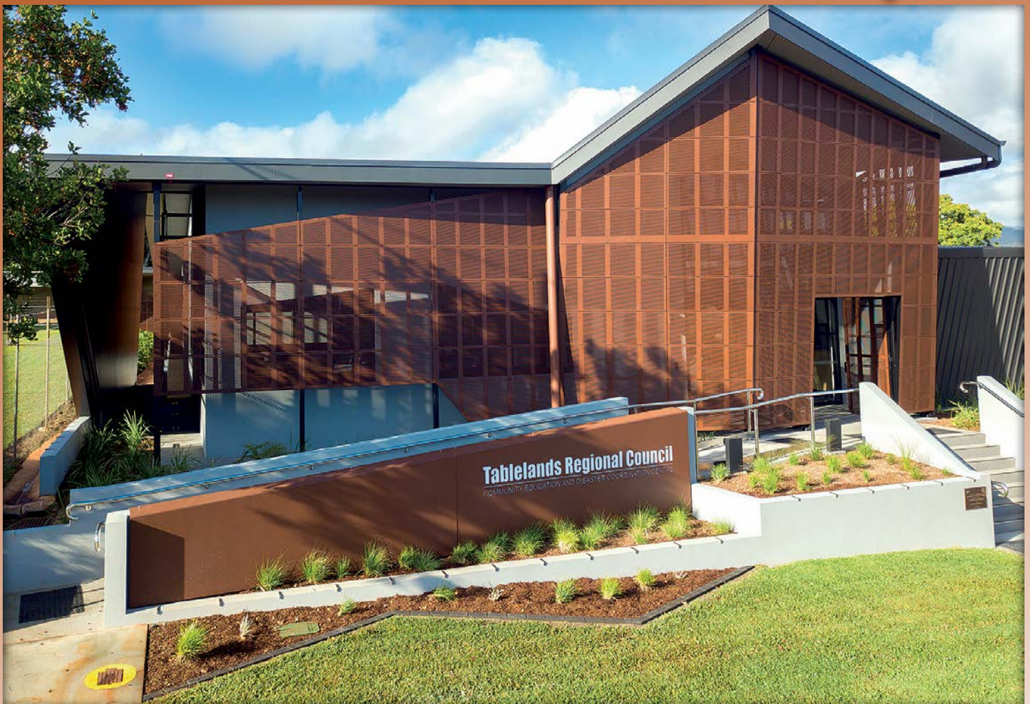
The newly opened Tablelands Regional Council Community Education and Disaster Coordination Centre at Atherton.
