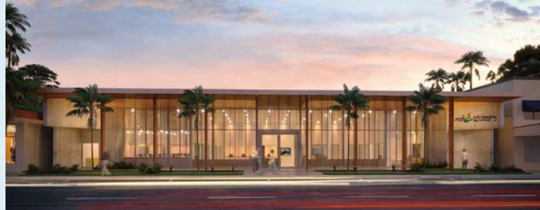
An administration building and local disaster coordination centre is under construction in Proserpine.
