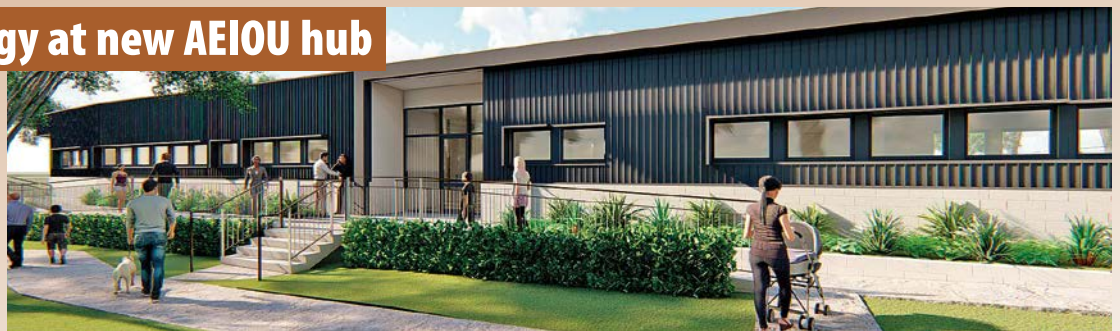
Purpose-built AEIOU centre is under construction.
