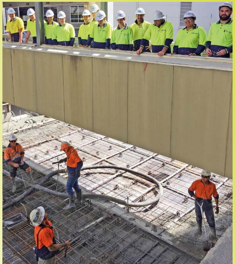
Hutchies' training students get a concreting presentation from Pro Concrete.
