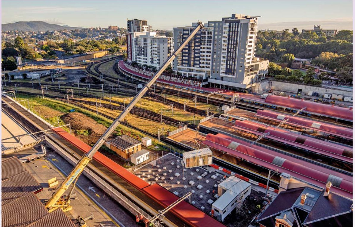
RIGHT: Demountable buildings were assets for the construction timeline.
