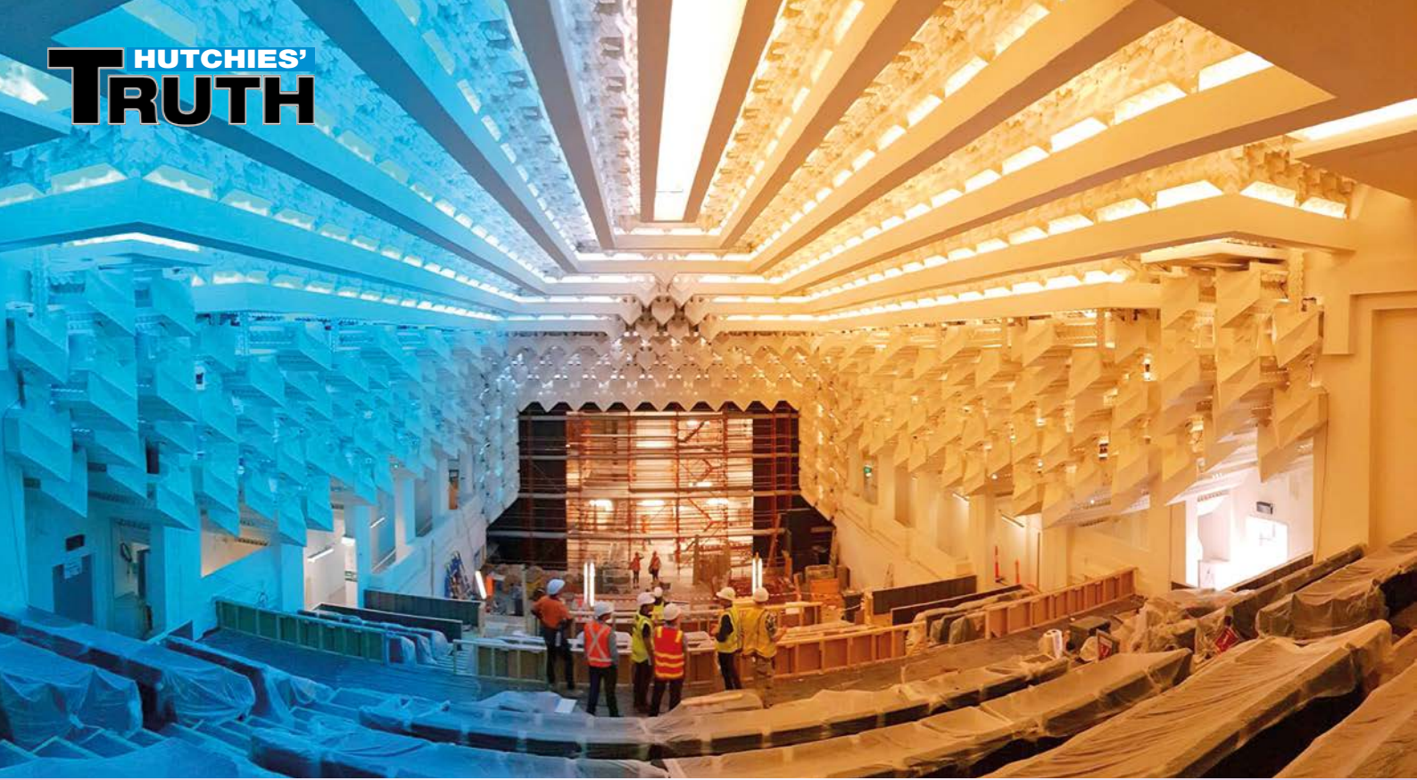
Work is nearing completion on RMIT's Capitol Theatre.
