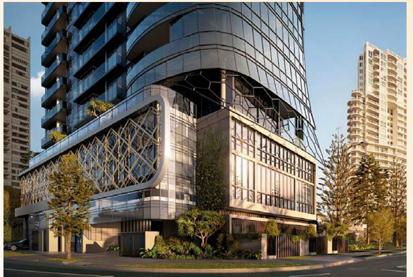
Elysian apartments minimised basement car parking area and cost with a mechanical parking system.
