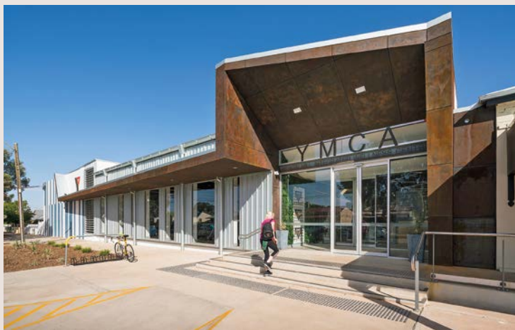
Newly completed YMCA Integrated Wellness Centre in Broken Hill
