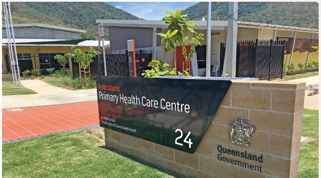
HUTCHIES has constructed a $12 million-plus medical facility on Palm Island. The new Palm Island Primary Health Care Centre includes consulting rooms, child and maternal health, and mental health facilities.
